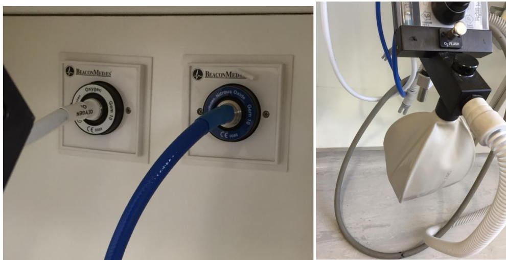
Figure. 5. Safety features of the Matrix MDMr N 2 O/O 2 Mixer machine for dental sedation. (a) Colour coding of tubings and (b) oxygen flush button and reservoir bag.
